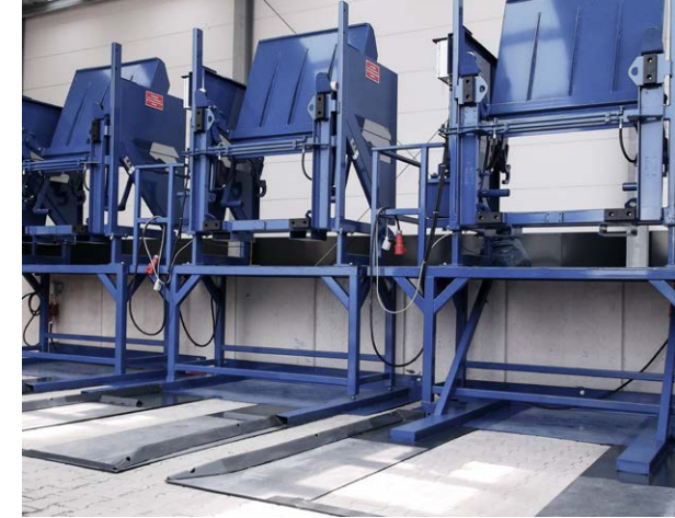
Ramp installation of static bin-lift devices
