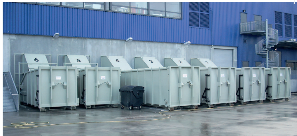
Transport containers at static compactor facility
