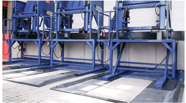
Ramp installation of static bin-lift devices
