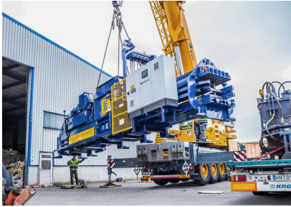
Installation of an AVOS 1810 B5-90/100
