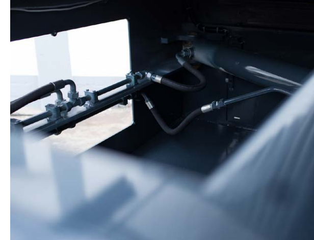
Large maintenance opening
