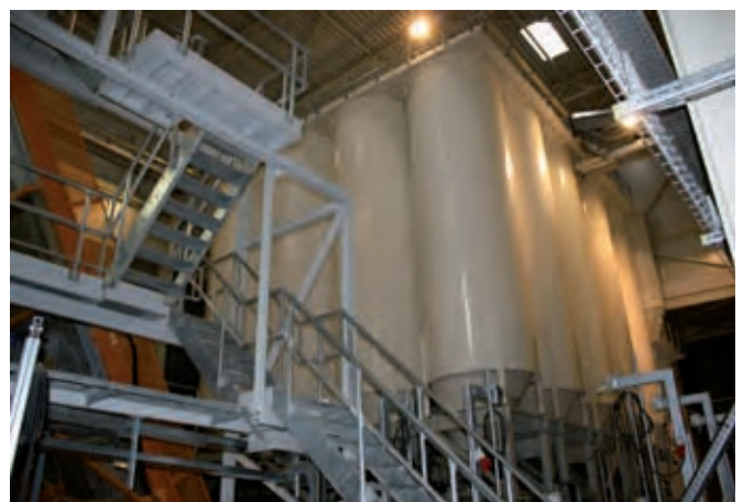
Distribution of aggregates to the 24 silos
