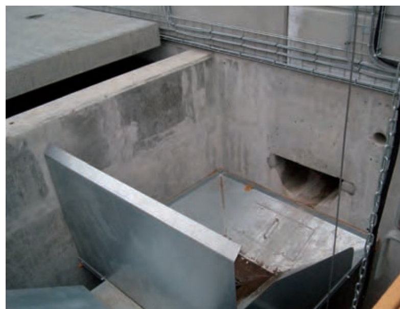
Gully to RWS plant transfer area
