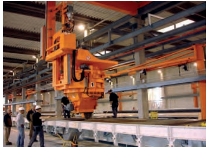
First concreting during the opening ceremony on 8/8/08 at 8.08 am
