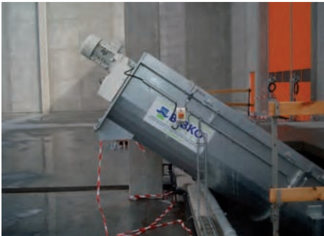
RWS delivery (during installation)
