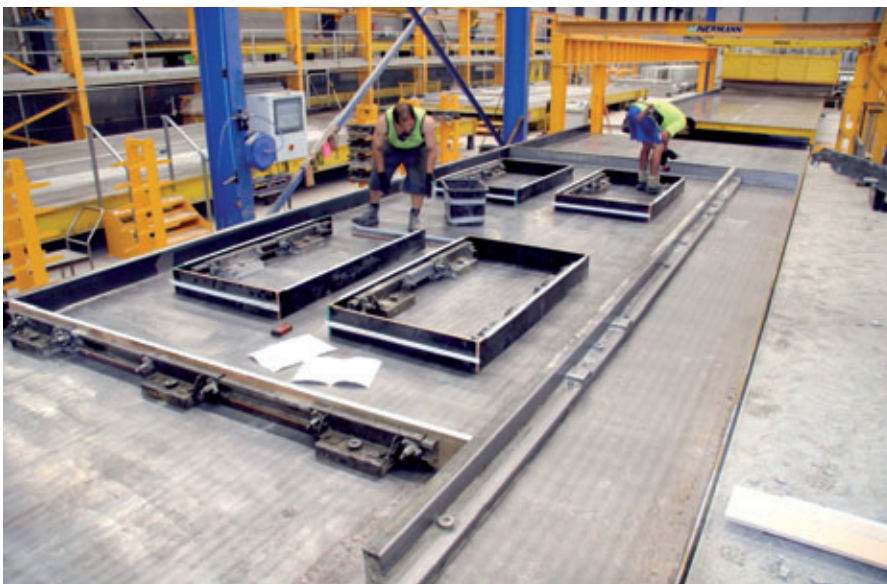
Manual formwork bay
