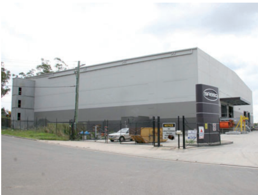
New production hall
