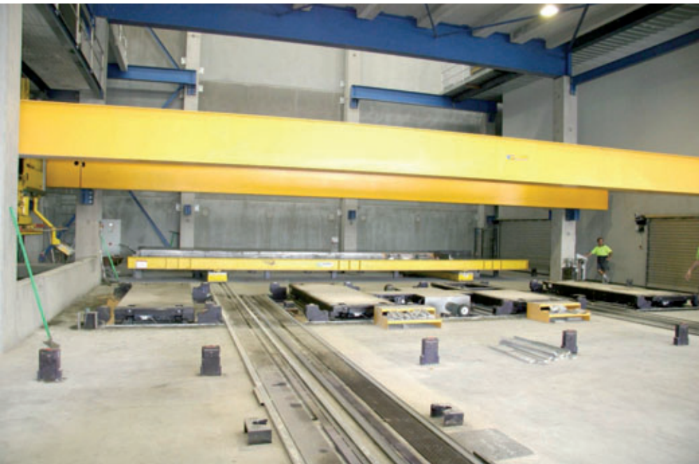
Transverse travel under concrete spreader and vibratory compactor
