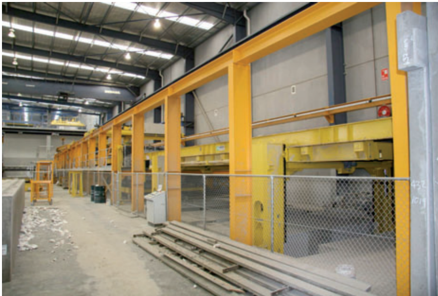
Precuring tunnel and smoothing bays
