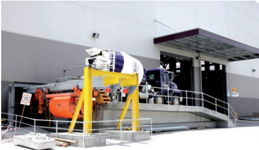
Filling the bucket conveyor with ready-mix trucks
