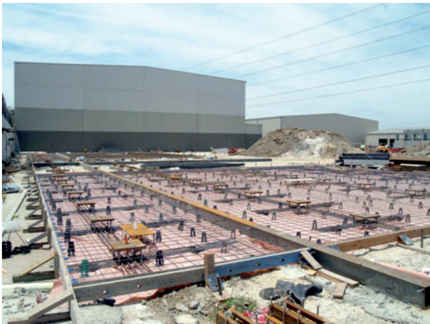
Groundwork for the new hall
