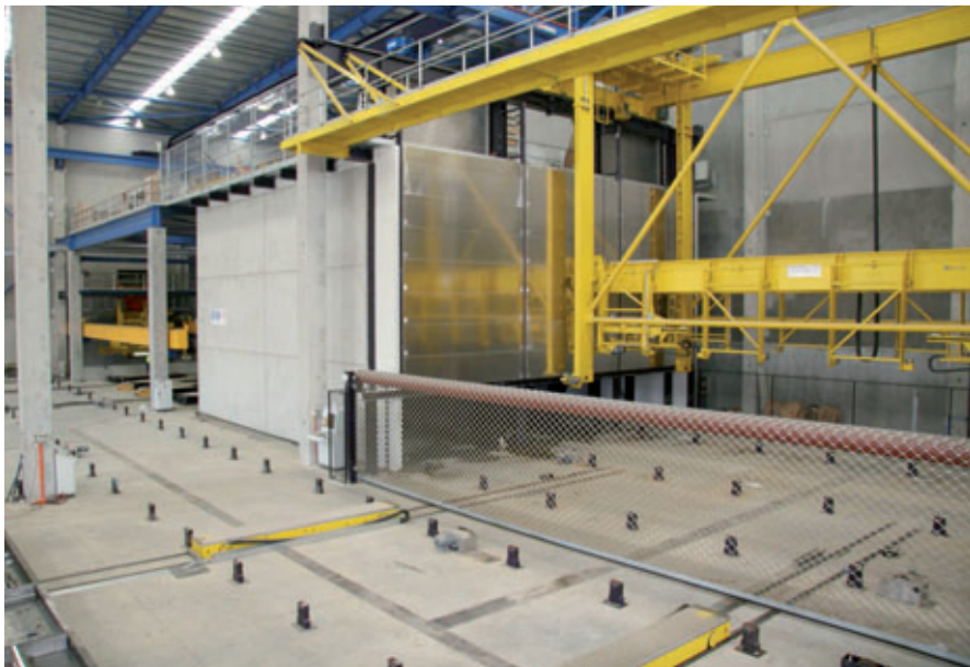
Curing chamber with storage and retrieval unit
