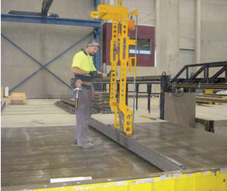
Formwork handling device
