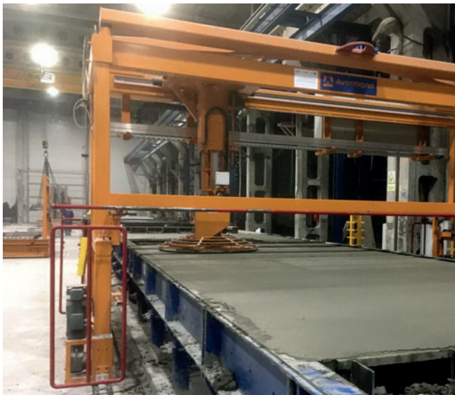
Power trowel during the smoothing process
