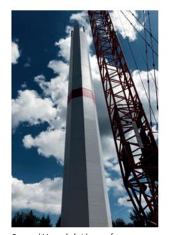
Patented Ventur hybrid tower for wind turbines
