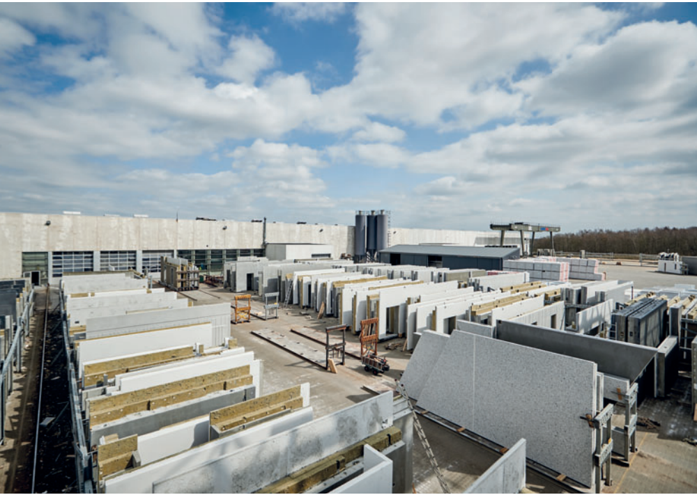
Fig. 2: View of the two production halls from above the open-air storage area; the central mixing system is in the middle
