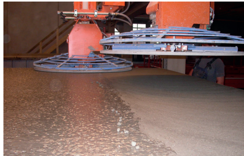
Abb. 6: Upper side post-treatment with power trowels
